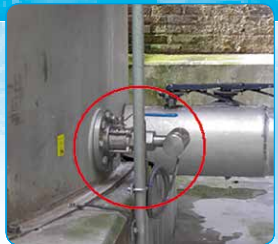
Level measurement in a large storage tank
